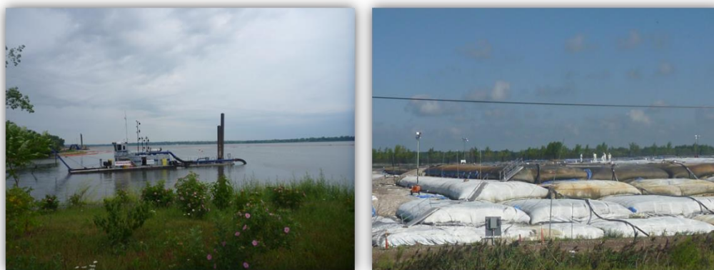
Dredging boat in Onondaga Lake and bags of dredged sediment in wastebed.
