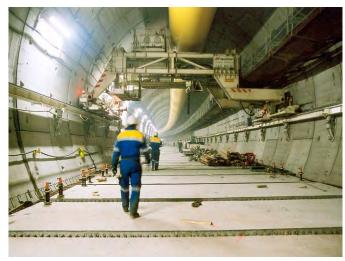
FIGURE 27: Paris A86 Tunnel – Installing Lower Deck
