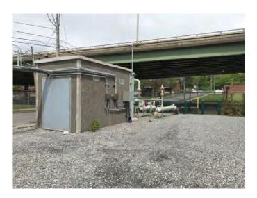
**FIGURE 4:** BFAS 1st Cut Gas House-12" Natural Gas Pipe Line at 600-800psi
