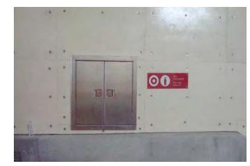
FIGURE 12: Stainless Equipment Cabinet for Fire Hose Valve and Extinguisher
