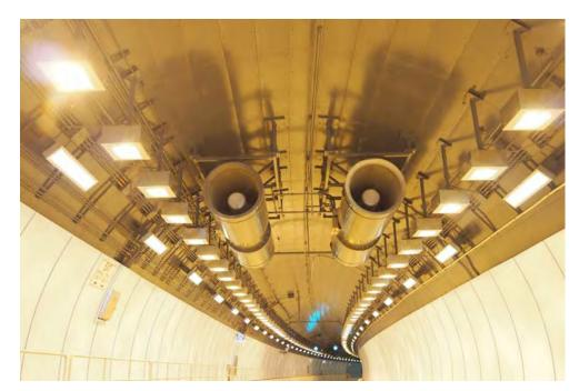
FIGURE 7: Single Bi-Level Tunnel with Jet Fan Instillation
