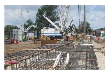
FIGURE 4: Rebar Cage for slurry wall, First Street Tunnel, Washington DC
