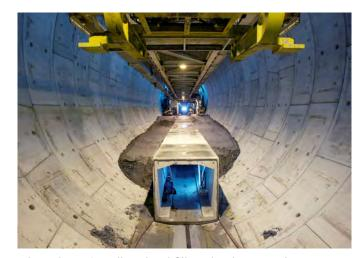
FIGURE 26: Installing backfill and utility corridor in Groene Hart Tunnel, Netherlands
