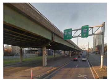
FIGURE 12: Low Headroom under Existing I-81 Viaduct
