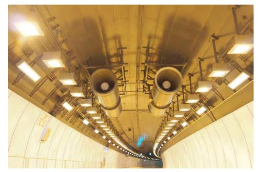
FIGURE 6: Twin Bored Tunnel with Jet Fan Installation
