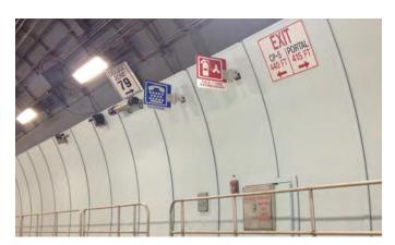
FIGURE 13: Example of Various Types of Signs Utilized in Road Tunnels to Identify Safety Related Features
