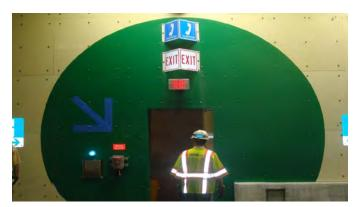
FIGURE 15: Photo showing egress opening, traffic barrier with angled interruption, painted board fireproofing, signage, and equipment cabinets
