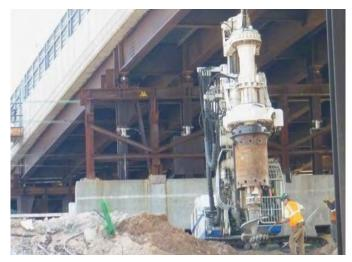
FIGURE 6: Secant Pile Wall Construction (23-ft vertical clearance), East Side Access, New York clearance
