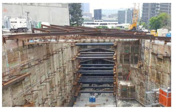
FIGURE 15: Soilder Pile and Lagging, 2nd and Hope Station, Metro Regional Connector, Los Angeles, Ca
