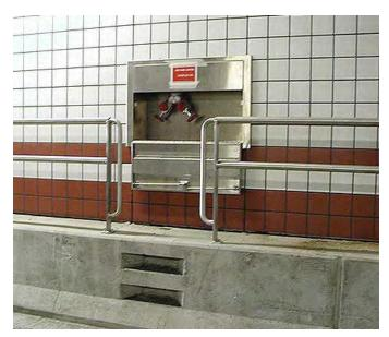
FIGURE 8: Typical Standpipe Hose Valve Cabinet
