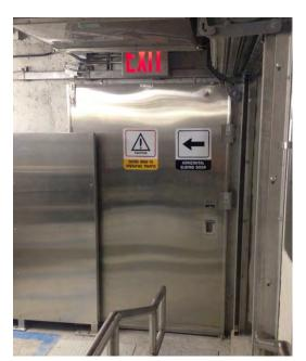
FIGURE 17: Stainless Steel Sliding Egress Door
