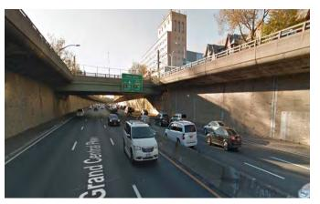
**FIGURE 19:** Depressed Highway with Cantilevered Almond Street
