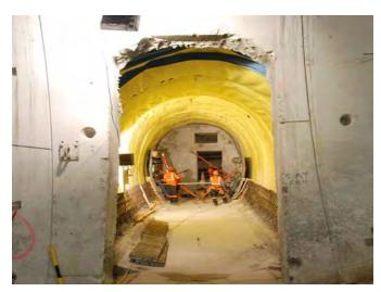
FIGURE 30: Waterproofing Membrane in Cross Passage (Port of Miami Tunnel)
