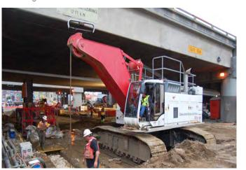
FIGURE 5: Slurry Wall Construction, 13 ft. 10 in overhead clearance
