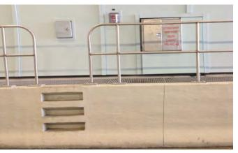
FIGURE 16: Photo Showing Raised Safety Walk in Concrete Traffic Barrier
