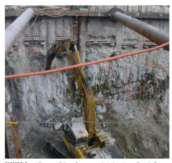
**FIGURE 3:** Secant Piles, Struts and tiebacks — South Ferry Station, New York
