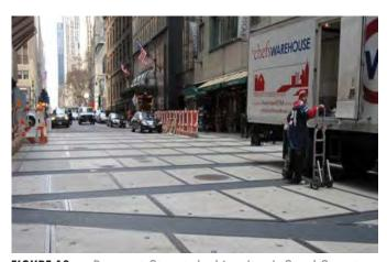
**FIGURE 13:** Pre-cast Street decking (top), Steel Street Decking (bottom) - 50th and 55th Streets Manhattan, NY
