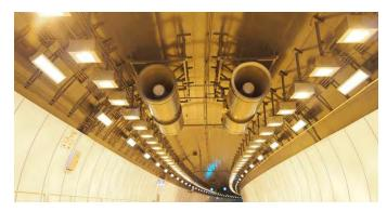
FIGURE 27: Single Bi-level Tunnel with Jet Fan Installation
