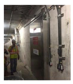
FIGURE 18: Construction Photo Showing Stainless Steel Sliding Egress Door inside Egress Corridor
