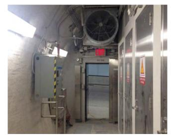
**FIGURE 21:** Cross Passage between Two Bored Tunnels Showing sliding door (open at far end), illuminated exit sign, equipment cabinets, pressurization fans, and emergency lighting fixtures (Port of Miami Tunnel)
